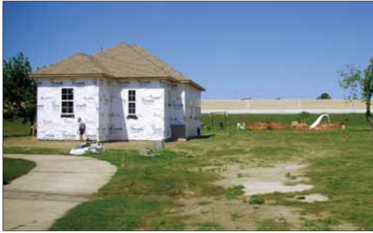
Left: A home in the lower Ninth Ward is rebuilt.
